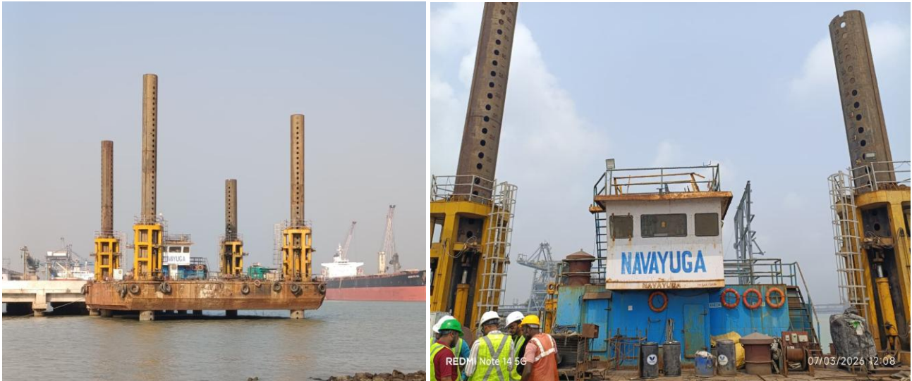
Fig-14 Deployment of Jackup Platform for Marine Geotechnical Investigation
