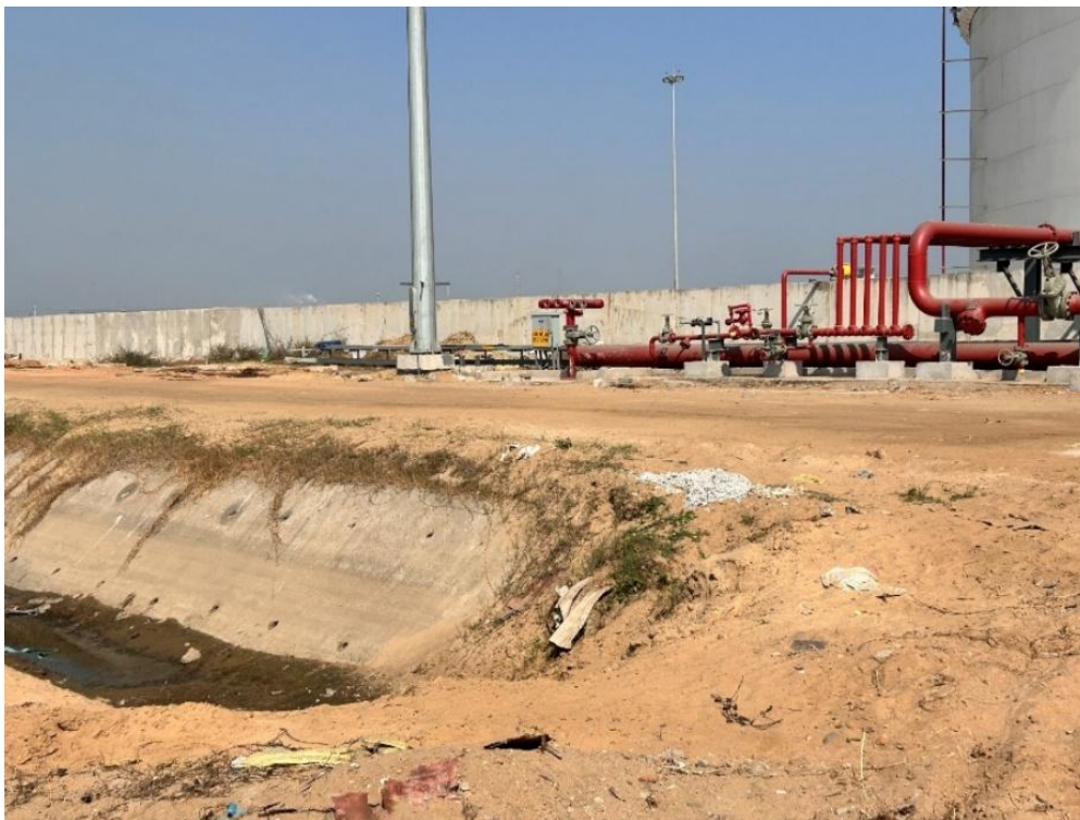
Figure 3: Road and Canal beside T-6 location
