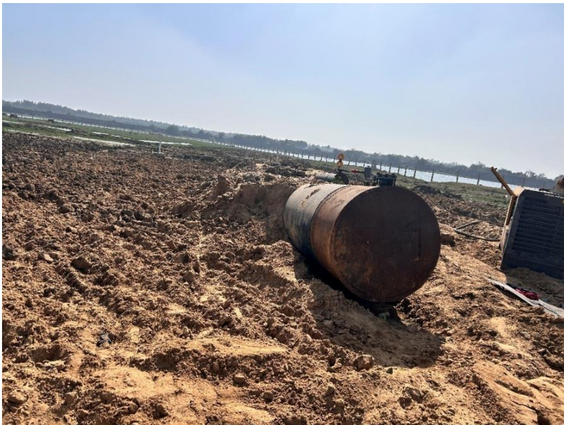
Figure 7: Start Point of HDD section of 4" ETP Pipeline
