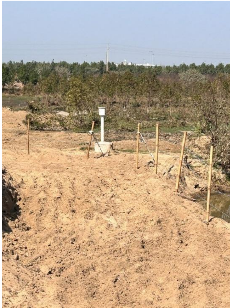
Figure 10: Pipeline Chainage Tower Before Forest Pipeline will be crosses the forest area through HDD.
