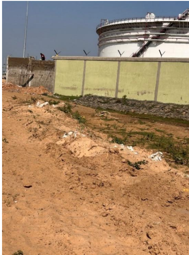
Figure 6: Boundary Wall and Outside Area of NRL COIT
