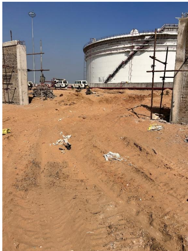
Figure 5: Boundary Wall of NRL COIT
